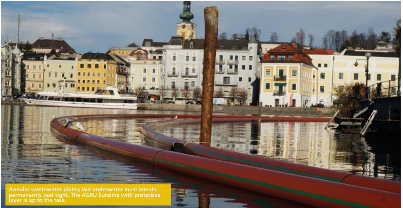
Annular wastewater piping laid underwater must remain permanently seal-tight. The AGRU Sureline with protective layer is up to the task.
