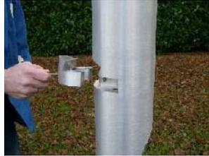
7. Hook the eye bolt with wedge onto your belt or place it on a toolbox and place your second hand onto the column.
