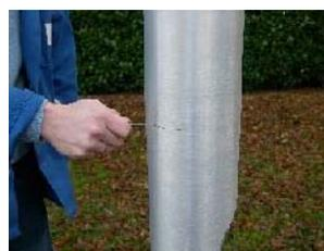
5. Use the supplied 'eye bolt' and place it into the threaded M6 hole.
