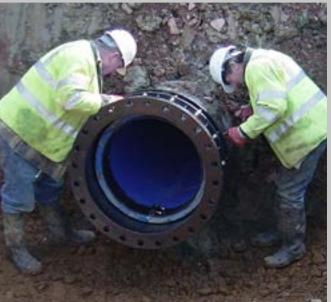
MULTIGRIP Country: United Kingdom Plant: drinking water hdpe pipeline Coupling: Multigrip flange adaptors *Connection of HDPE pipe with flanged valve*
