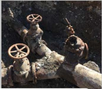
SPECIAL FITTINGS Country: Italy Plant: Water Treatment Plant Coupling: Special branch and Hawle valves *Replacement of valves of water treatment plant*
