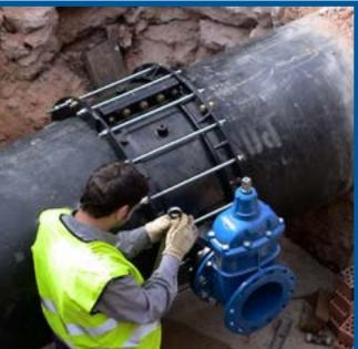
**SPECIAL FITTINGS** Country: Spain Plant: Aqueduct Coupling: Tapping tee coupling in two shells *hot tapping Duofit*
