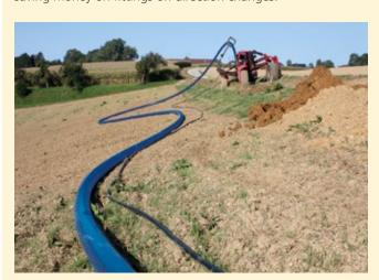
The coloured signal layer denotes the application - here a potable water line.
