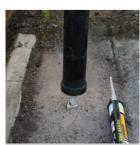
Step 4... Insert Bollard Assembly, twist in slowly
