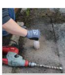
Step 2... Ensure hole throughly cleaned
