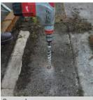
Step I... Drill hole using 24mm Masonary Bit
