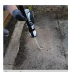
Step 3... Fill chemcial anchor flush with surface
