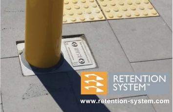
Further information on the RETENTION SYSTEM sockets for post installation is available at www.retention-system.com
